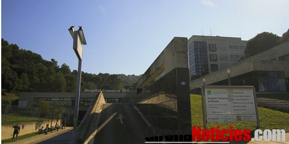
Hospital Comarcal Blanes
