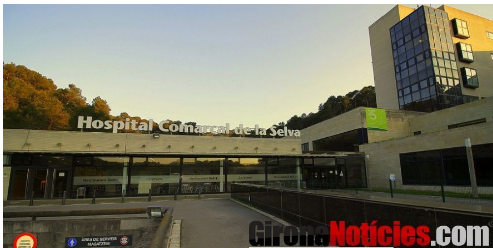
Hospital Comarcal Blanes
